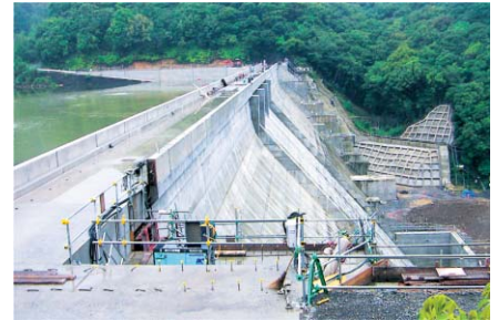
The Shimonohara Dam just prior to completion of the raising work
