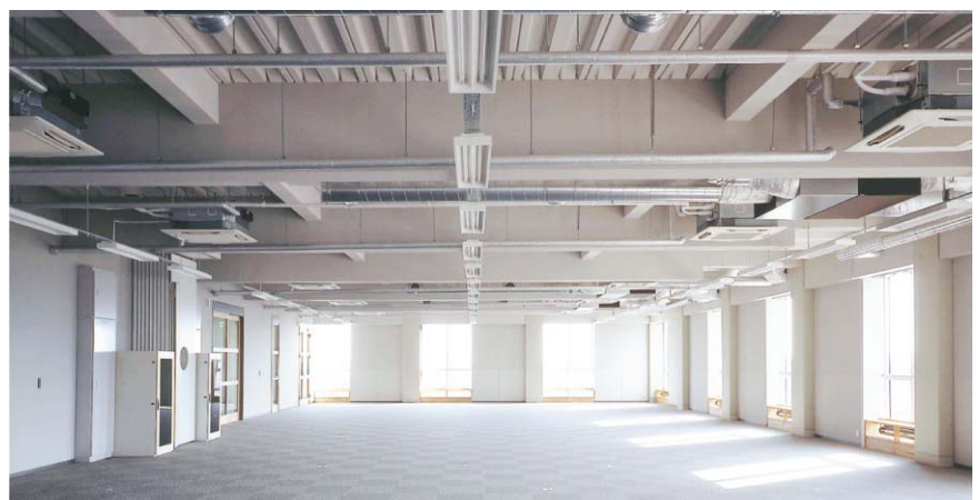
A school classroom constructed with the hybrid multi-tower construction method. The lack of support pillars offers an open space.
