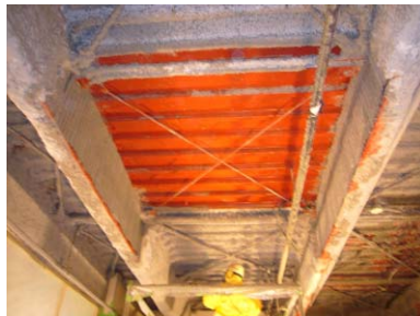
A ceiling after the asbestos removal procedure
