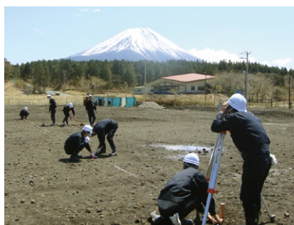
Civil Engineering Division's engineer trainees practice surveying.
