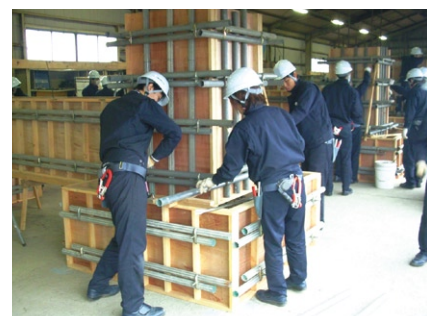
Building Construction Division's engineer trainees practice form work.
