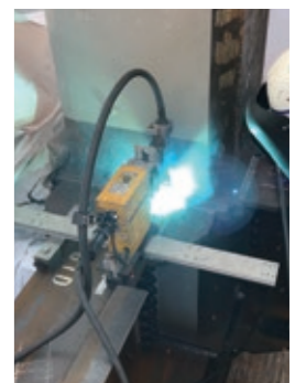
Ultra-narrow gap welding using a portable welding robot
