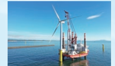
Construction for one of Japan's largest offshore wind farms
