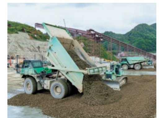
A 4 CSEL in use for embankment construction at Naruse Dam
