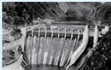
Japan's first high dam made of concrete, Ohmine Dam (Kyoto, 1924). Submerged in 1964 with the construction of the Amagase Dam
