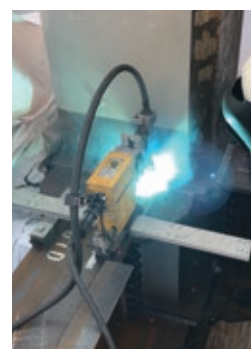
Ultra-narrow gap welding using a portable welding robot
