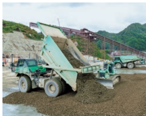
A 4 CSEL in use for embankment construction at Naruse Dam
