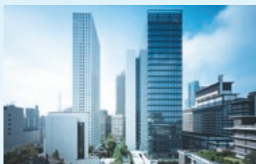
Toranomon Towers (2006), consisting of a 23-story leased office building and a 41-story residential condominium property on elevated ground in Toranomon, central Tokyo
