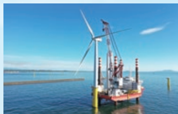
Construction for one of Japan's largest offshore wind farms
