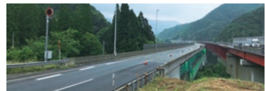
Kan-Etsu Expressway Anogawa Bridge, where deck slab renewal work will be carried out using the SDR system
