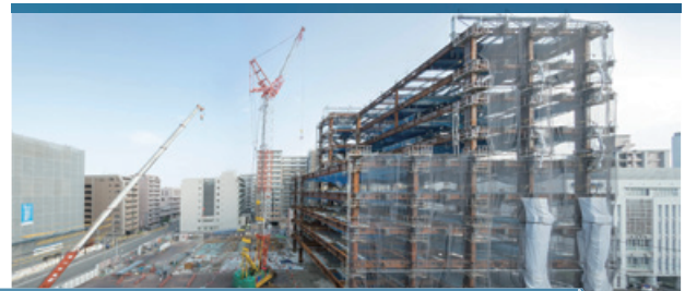
Construction State-of-the-art construction using smart construction
