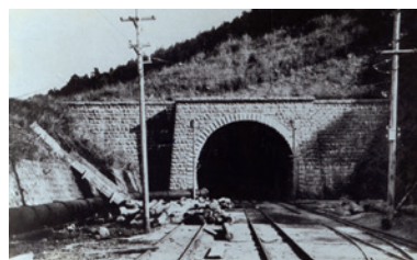
Tanna Tunnel (completed in 1934, Shizuoka)
