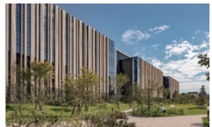
Chugai Life Science Park Yokohama (pharmaceutical-related facility)
