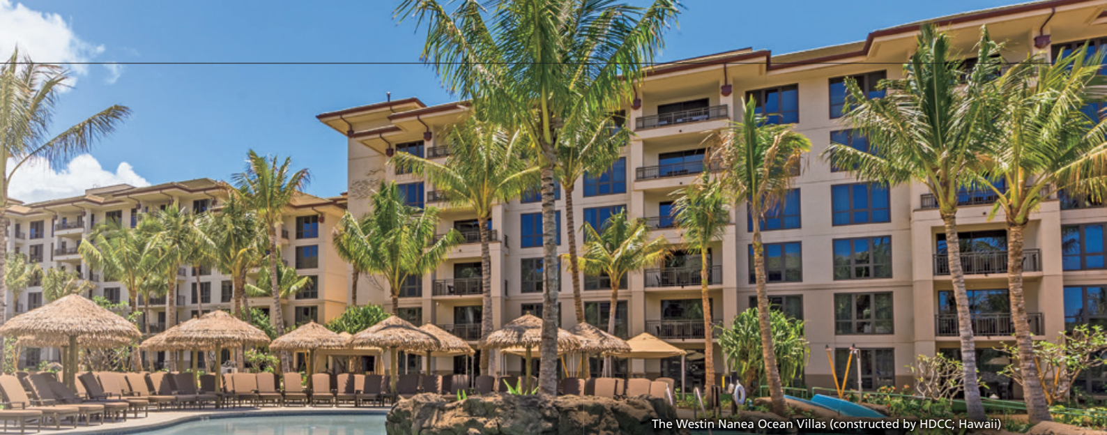
The Westin Nanea Ocean Villas (constructed by HDCC; Hawaii)
