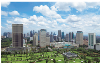
Senayan Square (development completed in 2015, Jakarta, Indonesia)
