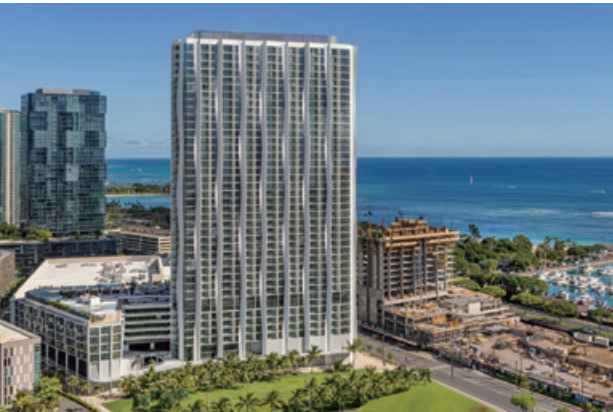
KŌ'ULA (constructed by HDCC; Hawaii)
