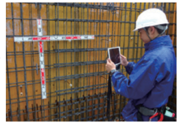
Reinforcement inspection by One Team
