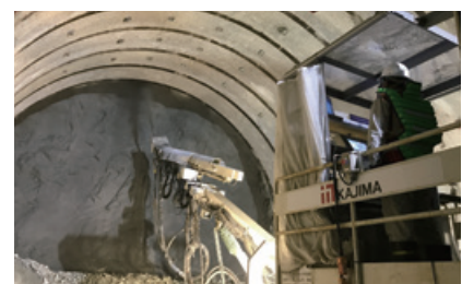
Automation of spraying operation (Kamioka Test Tunnel)
