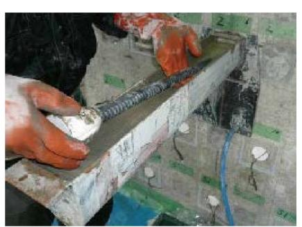
Insertion of a ceramic cap bar (CCb)
