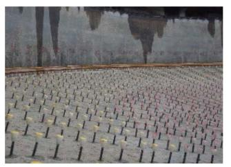
Reinforcement for a bottom plate of the gravity thickening tank
