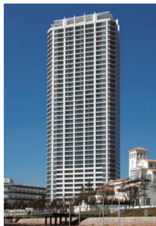
Super RC frame structure using ECC coupling beam
