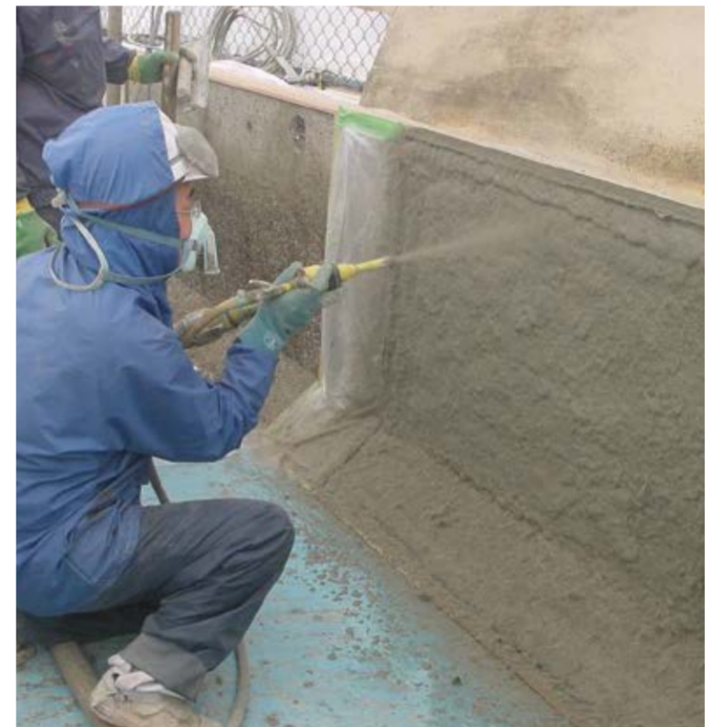
Example repair with direct spraying ECC shot
