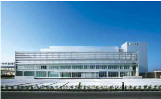
Solid Formulation Manufacturing Facility, Chugai Pharmaceuticals Fujieda Plant
