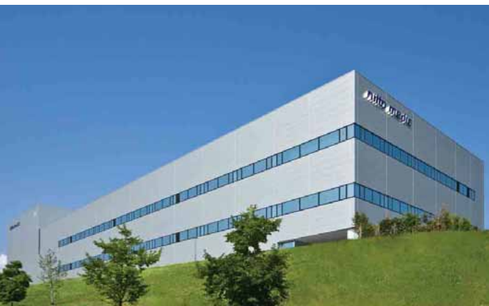
No. 3 Preparation Building, Nitto Medic Co., Ltd.
