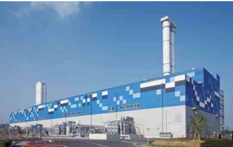
Shin-Nagoya Thermal Power Station Group No. 8
