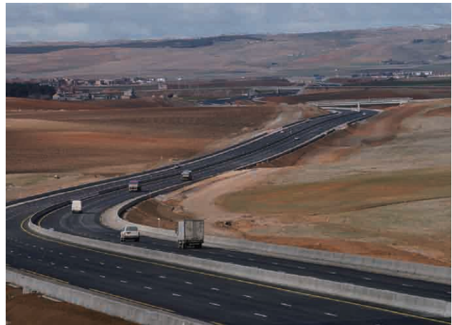
East-West Motorway, Algeria
