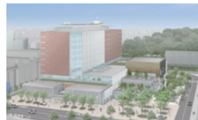
Machida City Government Office Building
