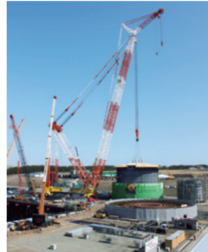
Installation using a large rotating crane
