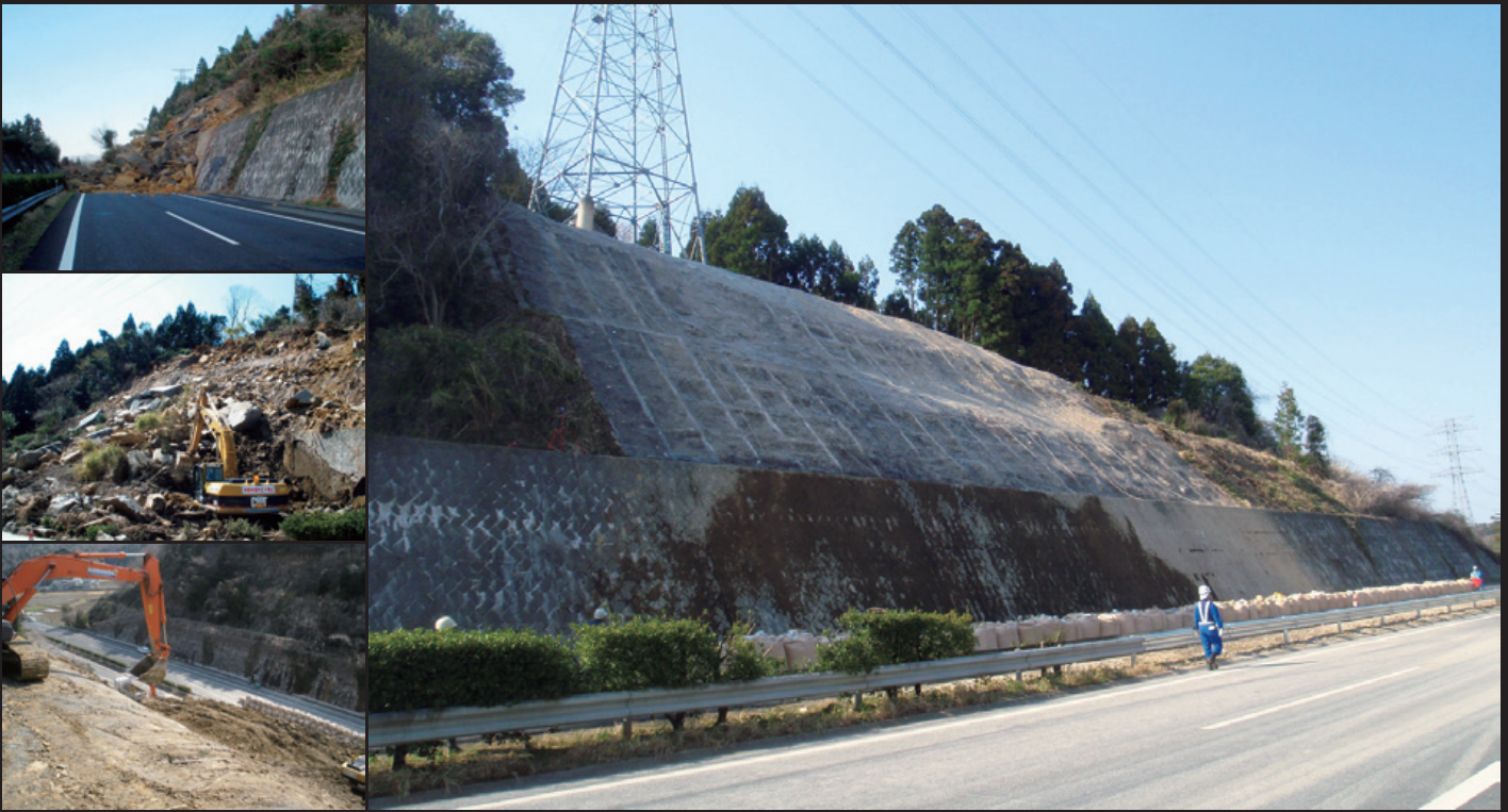
NEXCO East: Joban Expressway Iwaki restoration work—Service restored after 48 hours of work clearing approx. 4,000 m 3 of debris from a mudslide
