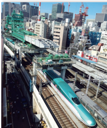
Viaduct being constructed above the Shinkansen lines
