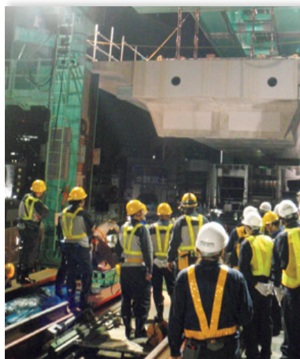
PC girders installed during nighttime work
