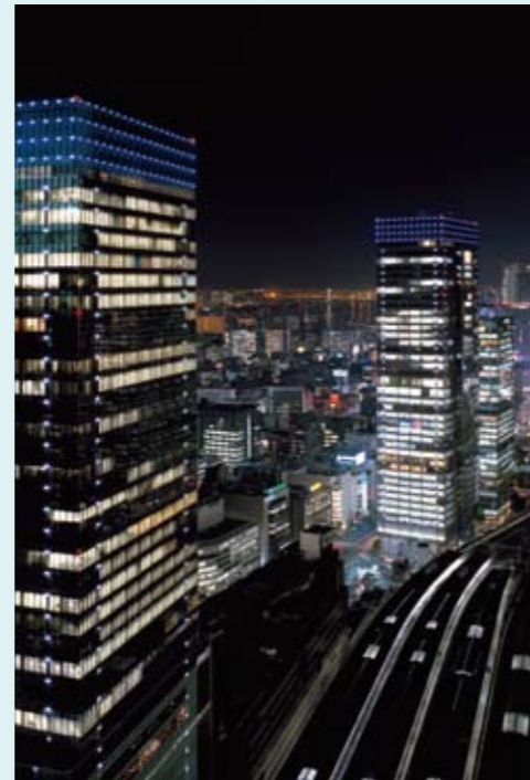
Redevelopment project for the Yaesu side of Tokyo Station
