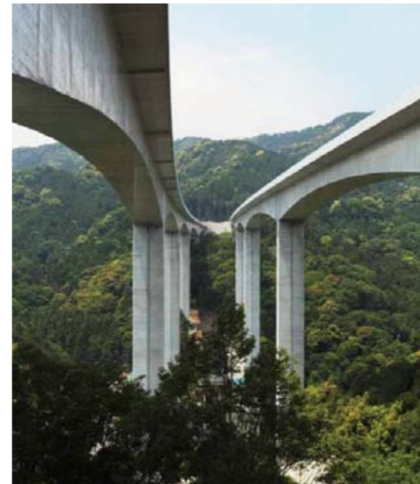
The New Tomei Expressway Sanagawa Bridge
