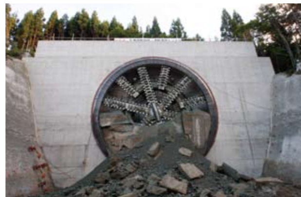
Tsugaru Yomogita Tunnel for the Hokkaido Shinkansen
