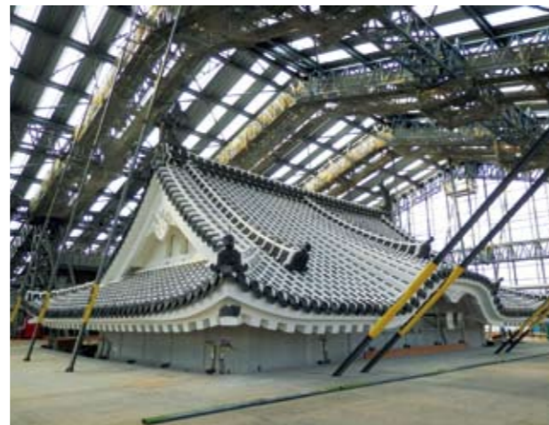
Restoration and repair work underway at Himeji Castle, a World Heritage Site
