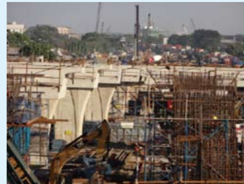
▲ Tanjung Priok Access Road (Sec. E2)
