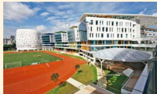
The New ITE College Central and ITE Headquarters
