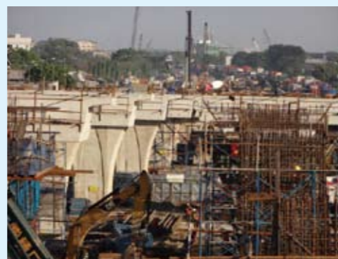
▲ Tanjung Priok Access Road (Sec. E2)
