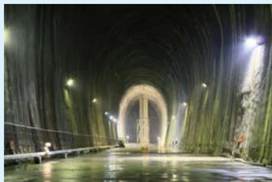
▲ International LPG Underground Plant in Kurashiki, Okayama Prefecture
