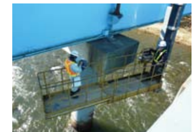
BM Star used during periodic inspections of this bridge
