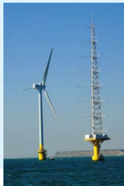
● Japan's first Offshore Wind Turbine and Met-mast conducted in the Pacific Ocean off Choshi City (NEDO* & Tokyo Electric Company)
