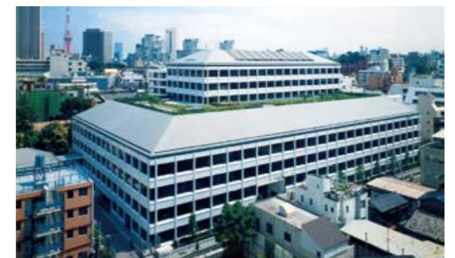
Kajima KI Building
