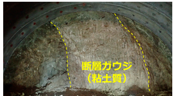
Fig.4 本坑の切羽写真 (Tunnel Face Picture of Main Tunnel)
