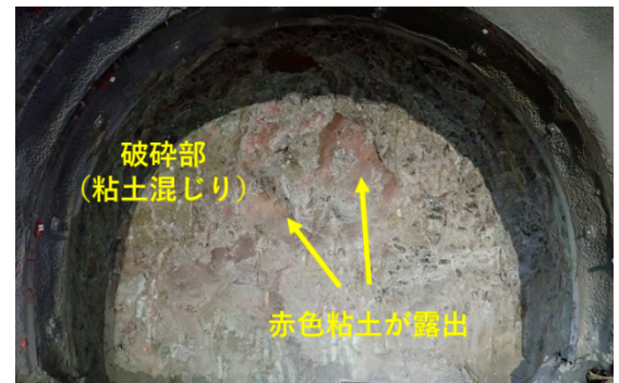
Fig.8 切羽写真 (TD.1,274m) (Tunnel Face Picture at TD.1,274m)
