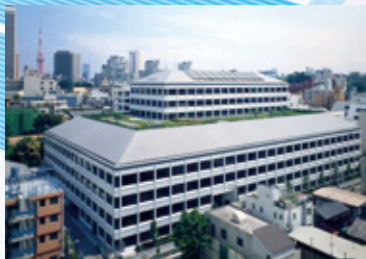
Kajima KI Building
