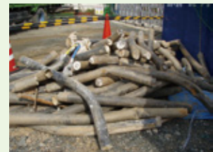
Removed tubes (old construction method)
