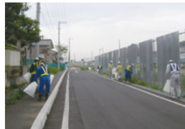
Monthly cleanup activities including all construction team members
