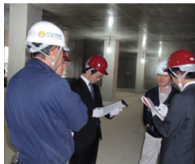
Answering students' questions while on a construction site tour
