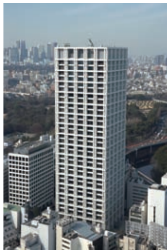
AKASAKA K-TOWER, a model of the future of large-sized tenanted buildings, aims to reduce CO 2 emissions by 40%
