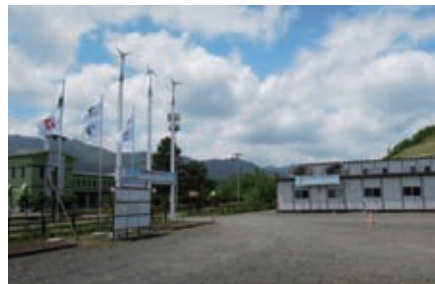
JV construction site office of Kitanomine Tunnel using photovoltaic (PV) panels and wind-power generation (Hokkaido Branch)
