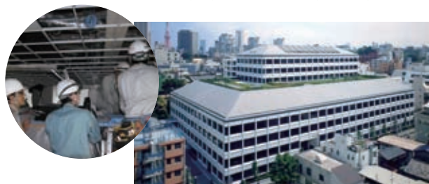
Renovation work (left) Kajima KI Building (right)
