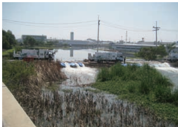
Japanese drainage pumps were very effective at the disaster sites.
