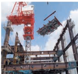
Lifting pre-assembled construction units that include beams, deck, and equipment
