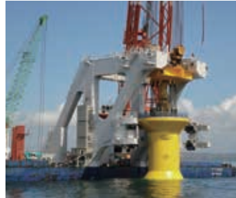
Installation of the wind turbine caisson
