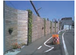
Construction site fence made from thinned wood from the village of Doshi, Minamitsuru, Yamanashi Prefecture (new building construction as part of redevelopment at the north entrance of Nagatsuda Station, Kanagawa Prefecture)
