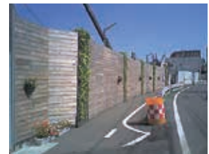
Construction site fence made from thinned wood from the village of Doshi, Minamitsuru, Yamanashi Prefecture (new building construction as part of redevelopment at the north entrance of Nagatsuda Station, Kanagawa Prefecture)
