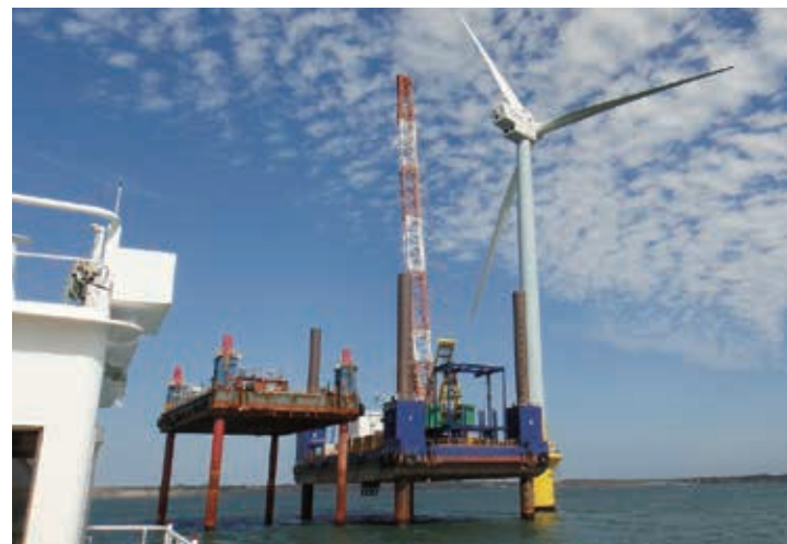
Installed offshore wind turbine using large self-elevating platforms
