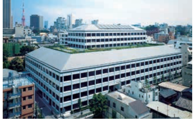
KI Building was transformed into a zero energy building
