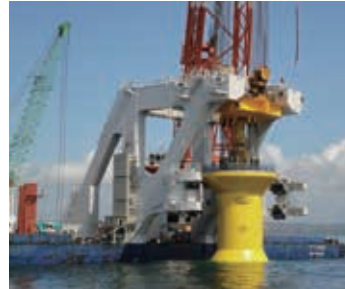
Installation of the wind turbine caisson
