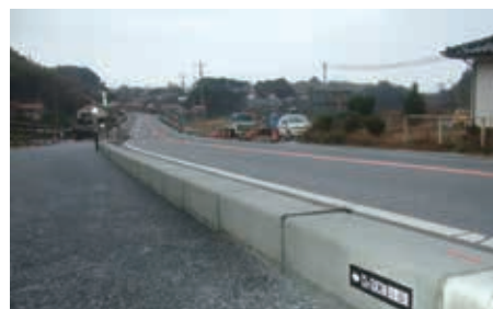
Hamada national highway constructed using CO 2 -SUICOM concrete
