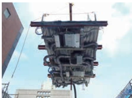
Lifting pre-assembled construction units that include beams, deck, and equipment
