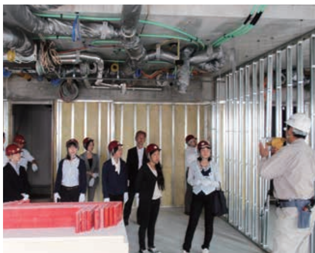
Tour of construction site for an ultra high-rise condominium
