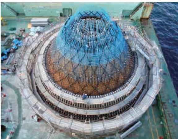
Rebar and PC steel wire used to make a foundation for an offshore wind turbine caisson
