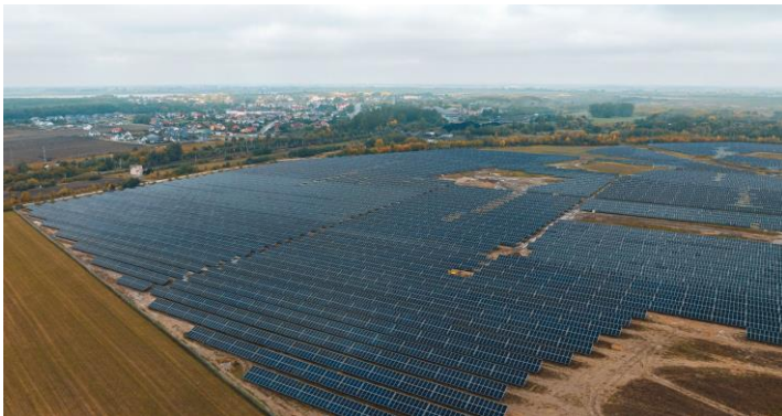
Genowefa Photovoltaic (Poland)
