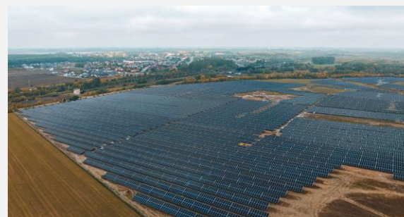
Genowefa Photovoltaic (Poland) Completed and delivered in Sep. 2023
