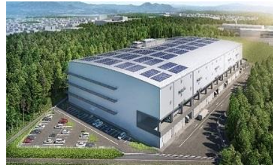
Kajima Tomiya Logistics Center (tentative name) (Miyagi Prefecture)
