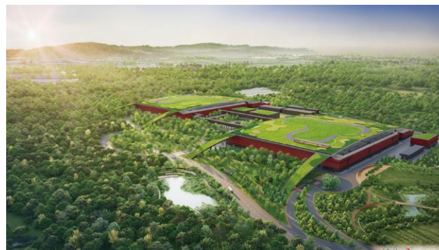
Rapidus IIM-1 plant Construction Project (Hokkaido)
