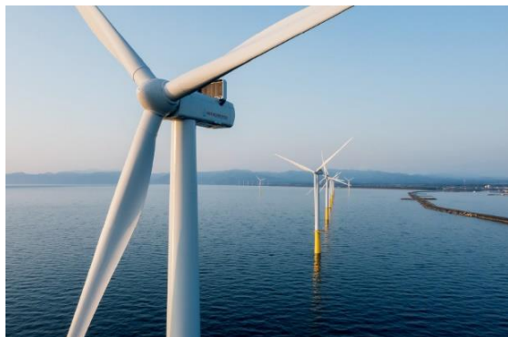
Offshore Wind Farms at Akita Port and Noshiro Port (Akita Prefecture)
