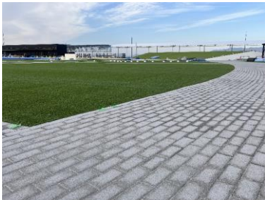
CO 2 -absorbing concrete used for venue paving (approx. 3,300 m 2 )
