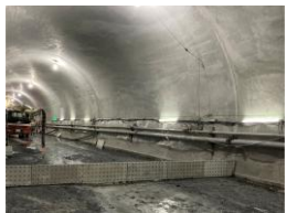
Installation of CO 2 -SUICOM formwork
