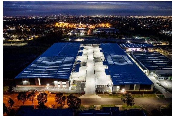
Broadfield Road distribution warehouse (Victoria, Australia)
