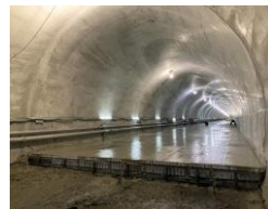
Completion of pouring
