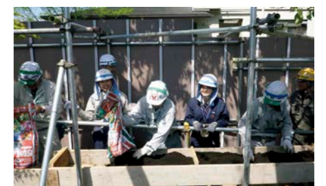
Preparing planters at a construction site for Kyoto Women's University
