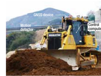
Networked bulldozer employing automation technology
