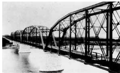
Aganogawa Railway Bridge
