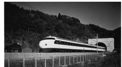
Shin-Tanna Tunnel for the Tokaido Shinkansen
