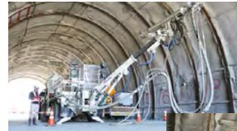
Demonstration of automated spraying in the mock-up tunnel
