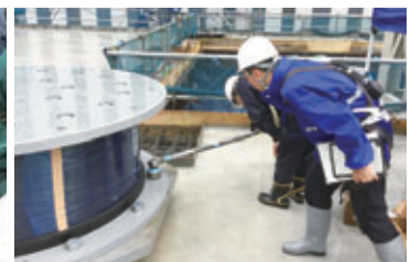
Confirming installation of a seismic base isolator
