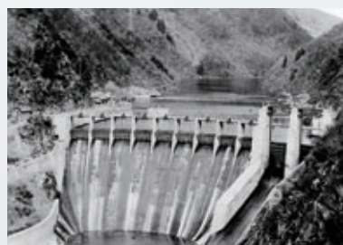
Japan's first high dam made of concrete, Ohmine Dam (Kyoto, 1924). Submerged in 1964 with the construction of the Amagase Dam.
