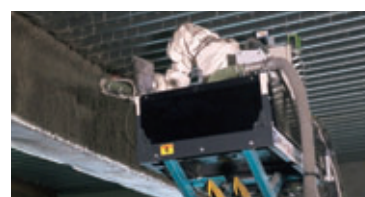
Construction using a fireproof coating spray robot
