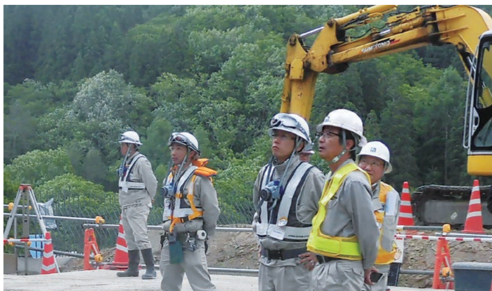
Hiroshi Shoji (foreground), General Manager of Tohoku Branch, observes construction at the Reconstruction Support Roads project.
