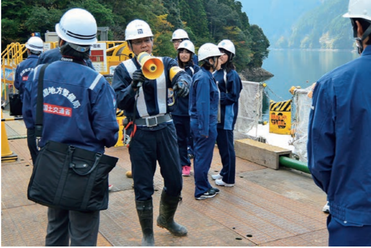
Thirty-one students from Anan College at the National Institute of Technology tour the local Nagayasuguchi Dam Renovation Project site.
