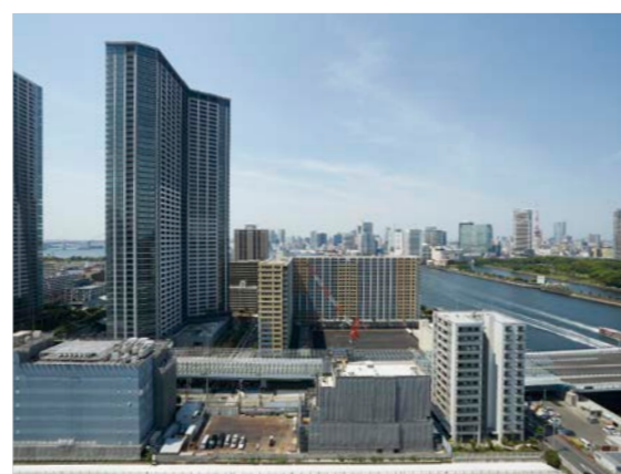
Kachidoki 5-Chome Redevelopment Project (Kachidoki The Tower)
