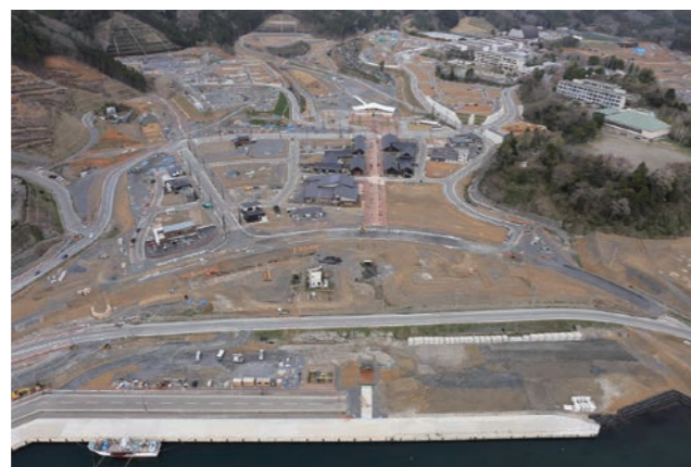
Onagawa Redevelopment Project
