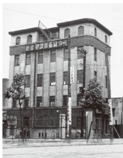
Kajima Technical Research Institute at its establishment in 1949
