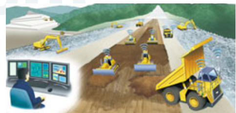
Commands are issued to automated heavy machinery from the control room
