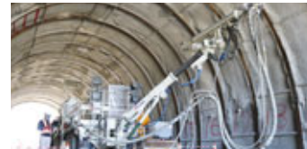
Demonstration of automated spraying in the mock-up tunnel
