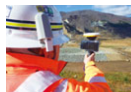
CIM model confirmation onsite using the handheld monitor
