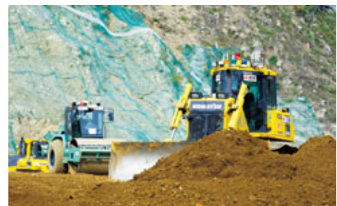
Core material construction for the Koishiwara Dam
