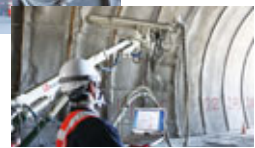
Demonstration of automated spraying in the mock-up tunnel
