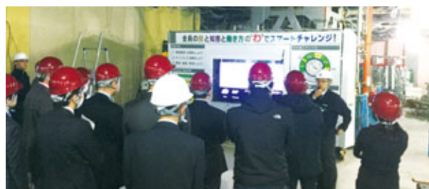
Construction site tour of Kajima Fushimi Building (tentative name)
