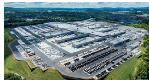
UPS Middletown (Pennsylvania)
