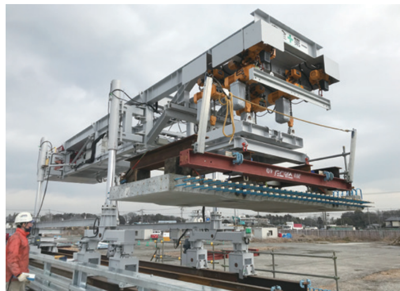
SDR System demonstration test. Machine to install precast slab
