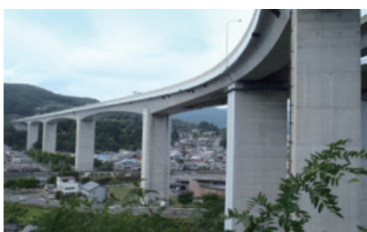
Nagano Expressway Okaya Viaduct (infrastructure renewal)
