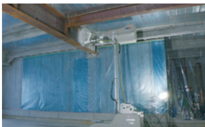
Fireproof coating sprayer robot (smart construction technologies)
