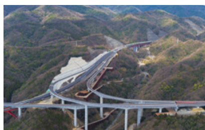
Hanwa Expressway Onoyama Viaduct (infrastructure renewal)
