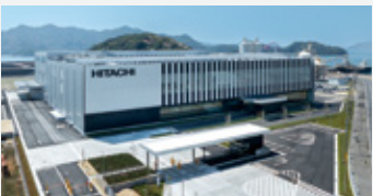
Hitachi High-Tech new manufacturing facilities in Kasado area
