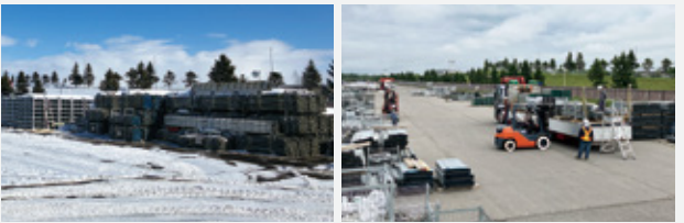
Temporary storage and sorting yard for temporary materials for the construction project of Rapidus IIM-1
