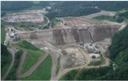
The Naruse Dam under construction
