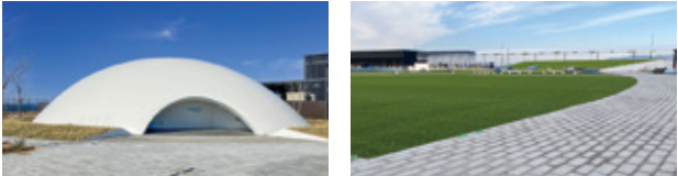
CUCO-SUICOM Dome (Sustainability Dome) completed CO2-absorbing concrete used for venue paving (approx. 3,300 m²)
