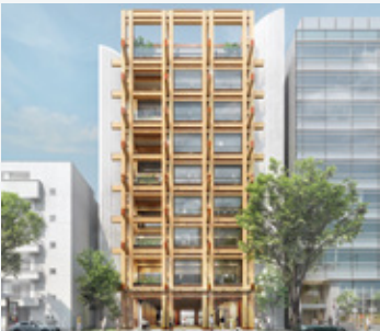
Exterior of the new Tohoku Branch building One floor underground, nine floors above ground. Wooden (seismic-resistant structure) with partial steel framework. Total floor area 8,872 m 2 Demolition work began in June 2025 and new construction work is scheduled to begin in FY2026 and end in FY2028
