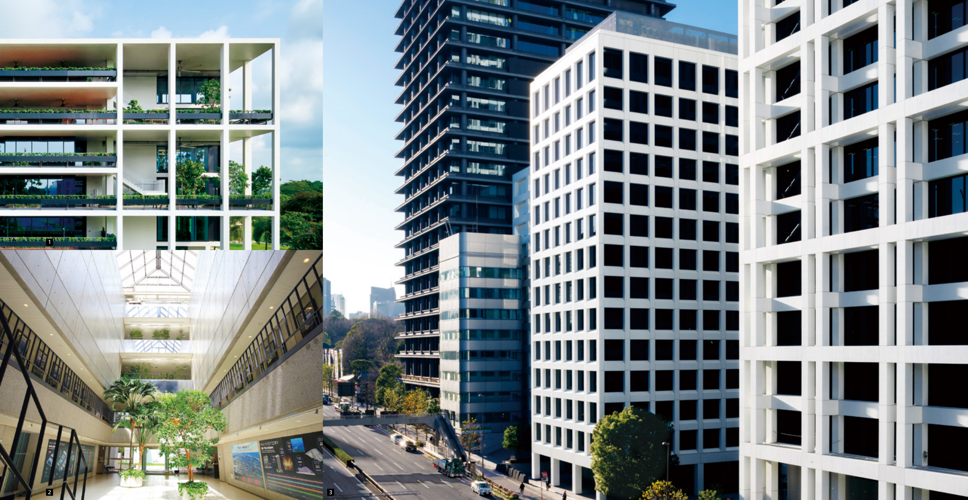
1: The GEAR (Singapore); 2: Kajima Technical Research Institute, Nishichofu Complex (Tokyo); 3: Kajima Head Office Buildings (Tokyo)
