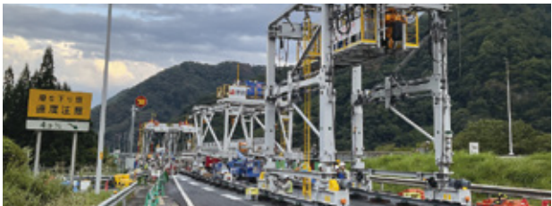
Shortened the deck replacement period by approximately 67% on the Anogawa Bridge deck replacement project on the Kan-Etsu Expressway (Gunma Prefecture—Niigata Prefecture)
