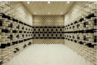
Renovated high-performance anechoic chamber
