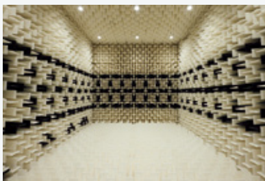
Renovated high-performance anechoic chamber
