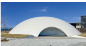
CUCO-SUICOM Dome (Sustainability Dome) completed
