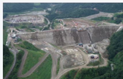
The Naruse Dam under construction
