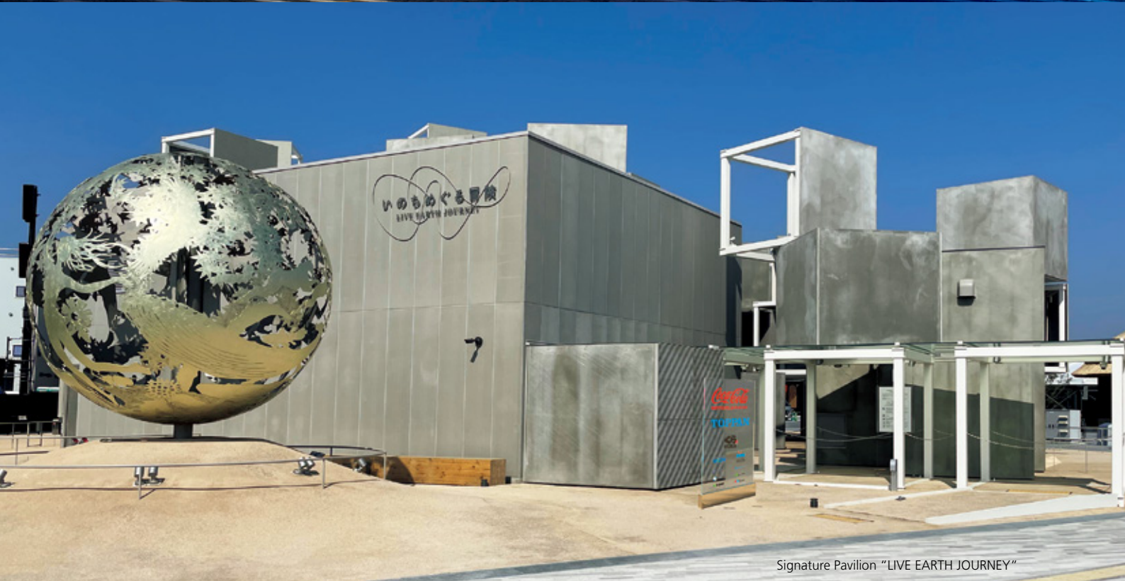
CUCO-SUICOM Dome (Sustainability Dome)
