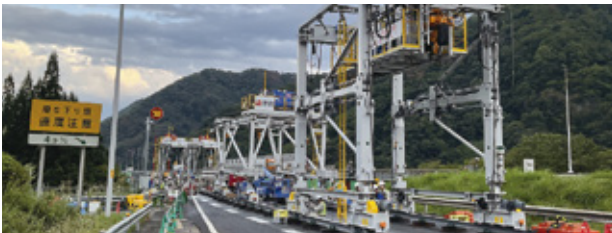
Shortened the deck replacement period by approximately 67% on the Anogawa Bridge deck replacement project on the Kan-Etsu Expressway (Gunma Prefecture—Niigata Prefecture)
