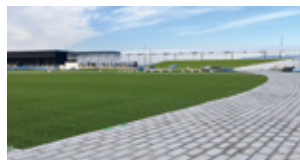
CO 2 -absorbing concrete used for venue paving (approx. 3,300 m 2 )
