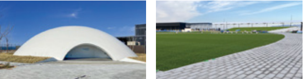
CUCO-SUICOM Dome (Sustainability Dome) completed CO 2 -absorbing concrete used for venue paving (approx. 3,300 m 2 )
