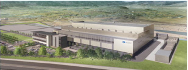
Construction of a new KOSÉ Corporation factory in the Minami Alps (Yamanashi Prefecture)
