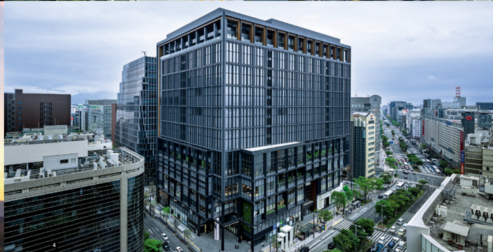
1: Victoria Place at Ward Village (U.S.); 2: KALOC TOMIYA (Miyagi); 3: Kawauchi Onitaroyama Wind Farm (Fukushima); 4: ONE FUKUOKA BLDG. (Fukuoka)
