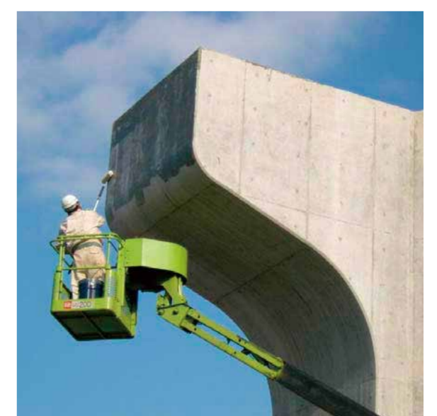
Application of Magical Repeller by using a roller
