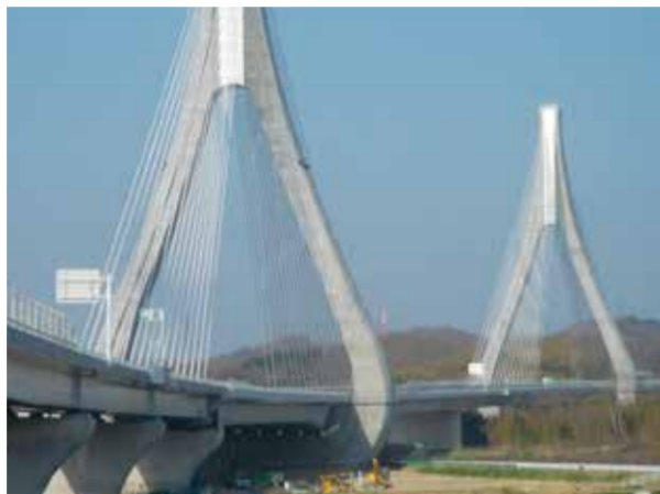
An examples of concrete structure
