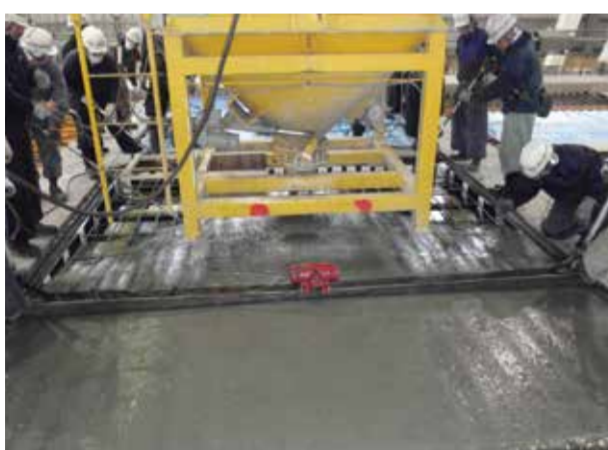
Placing of SUQCEM
