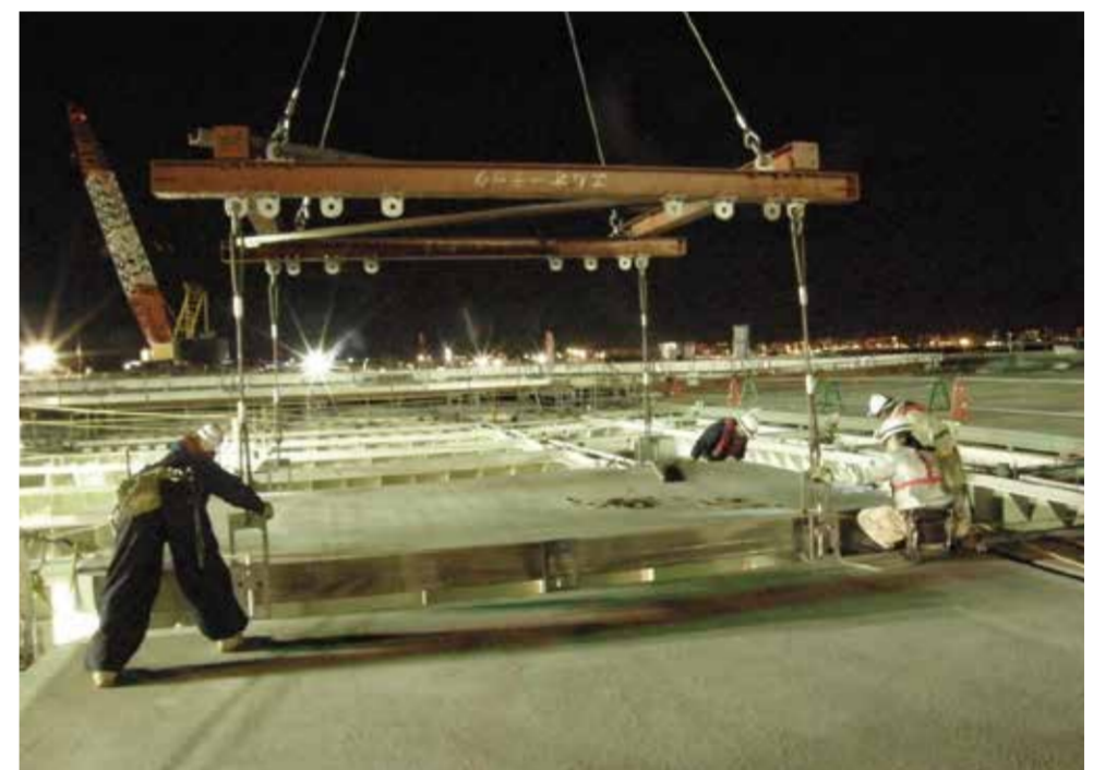
Installation of the SUQCEM floor slabs
