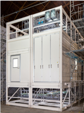
KaMoS® (Kajima Modular Facility System) A new modularization technology for biopharmaceutical manufacturing facilities
